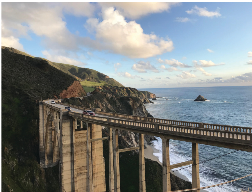
The Bixby Creek Bridge / Darwin Luna
